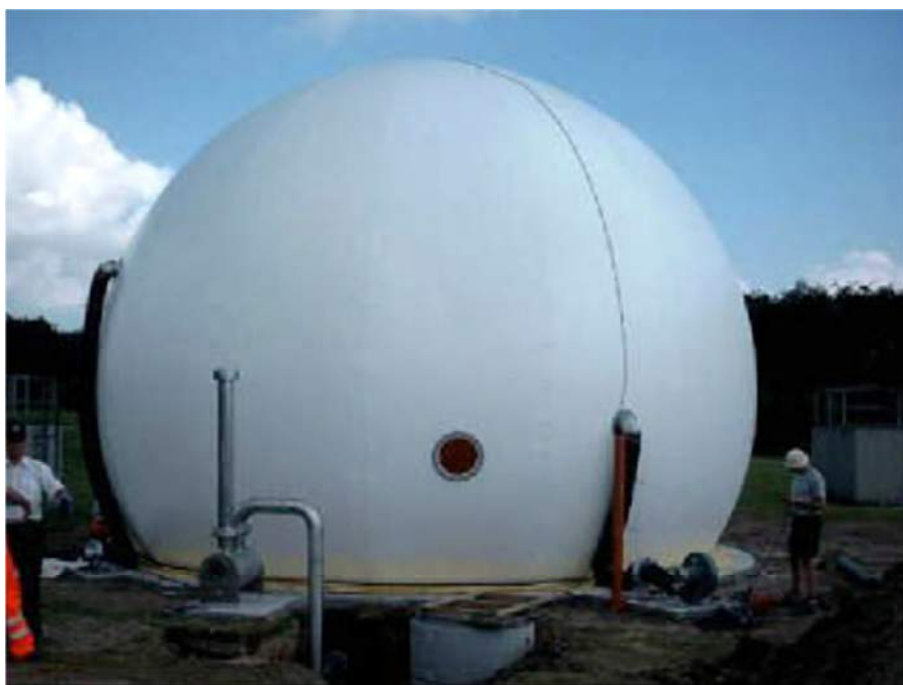
Figure 14: Gas storage with safety device
